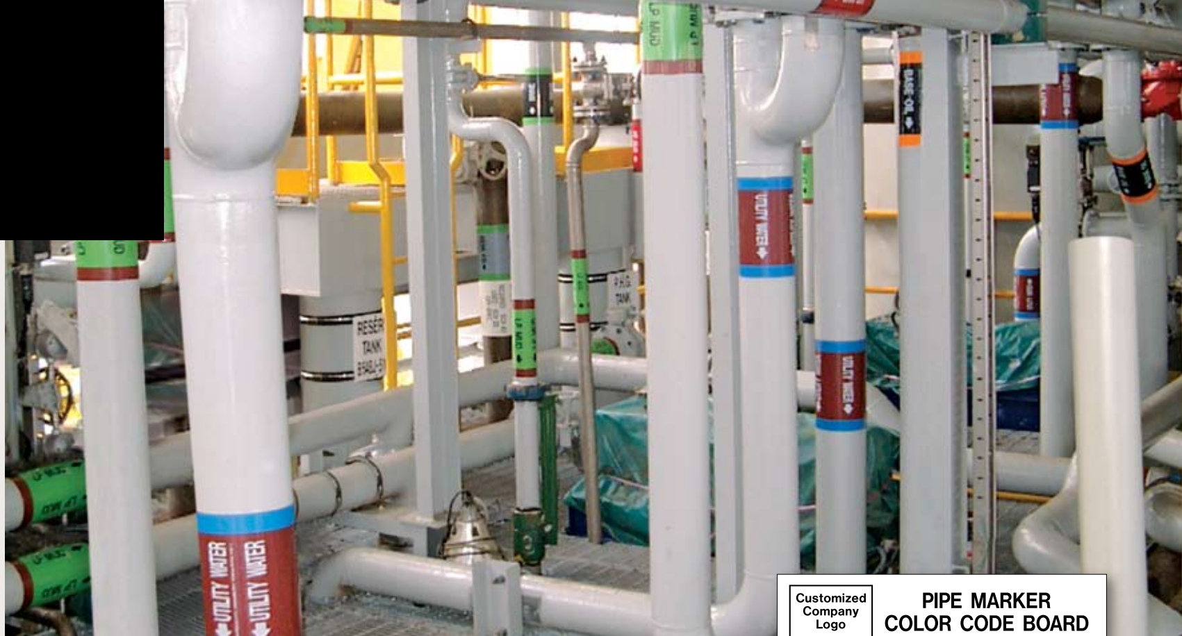
Typical pipe marker installation
